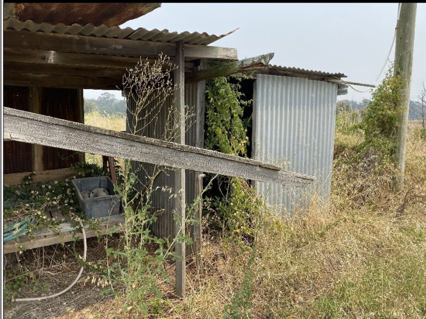
PHOTO 12: LOT L57 - SHOWING PRESENCE OF ASBESTOS SHEETING SOUTH OF SHED
