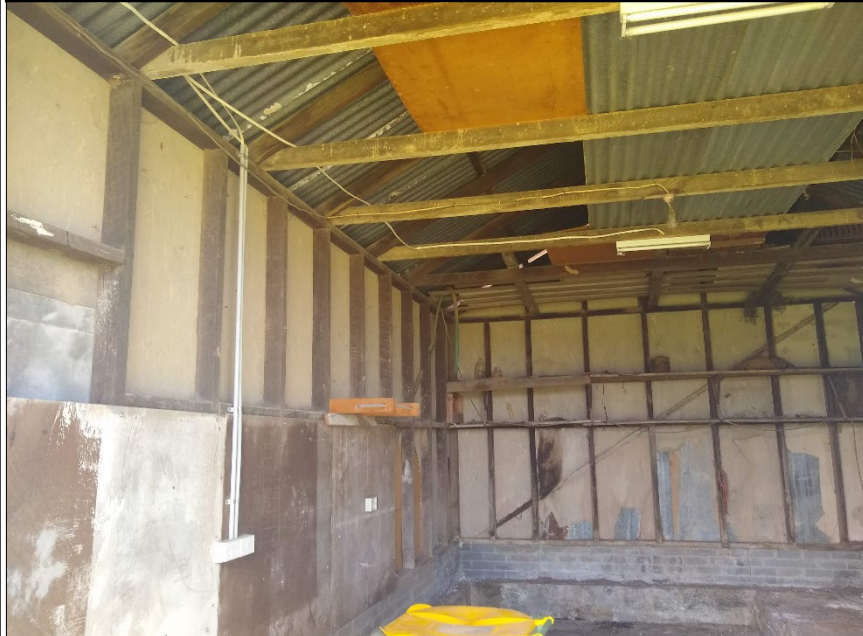
PHOTO 59: LOT 74B - SHOWING SHED WITH DAMAGED SUSPECTED ASBESTOS CONTAINING MATERIAL WALLS
