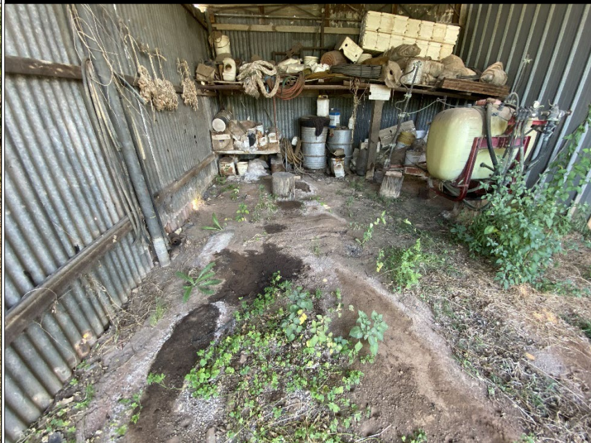
PHOTO 48: LOT L1 - SHOWING EXPOSED POTENTIAL ACM PIPE ADJACENT SHED
